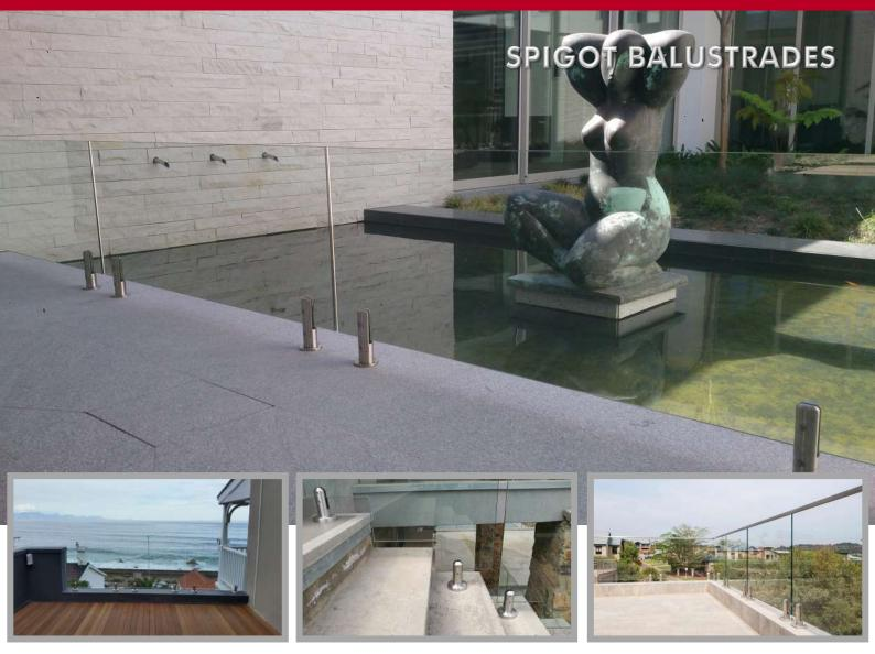
This system is the epitome of style and architectural elegance. The glass is clamped into a Stainless Steel or Aluminium, purpose made bracket (Spigot) which is mounted at the bottom on top of a support structure e.g. a concrete slab. Different shapes and designs of spigots are available for you to choose from.
